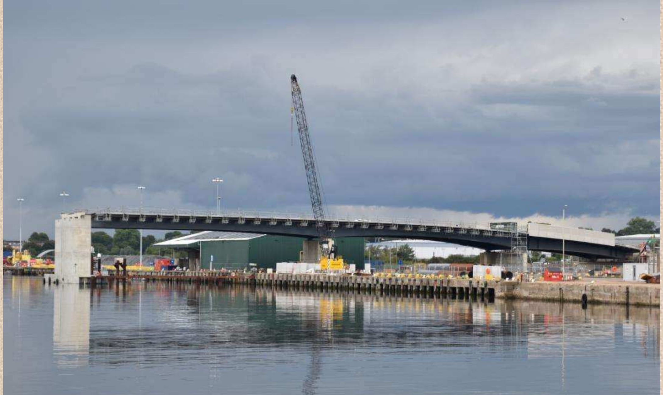
LW5 – Gull Wing Bridge North
