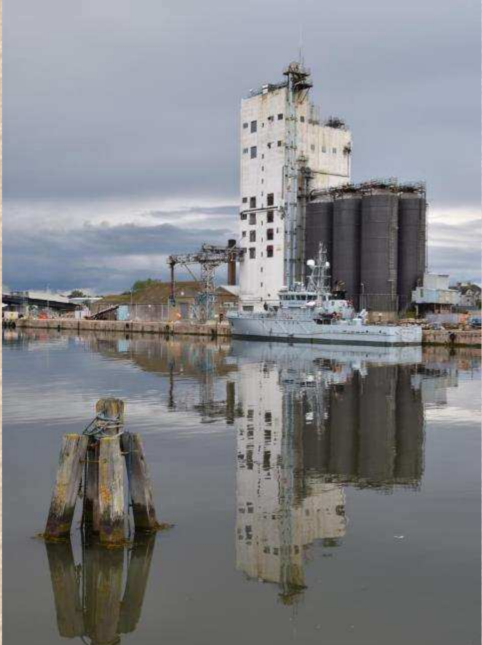
LW2 – Lowestoft Grain Silo
