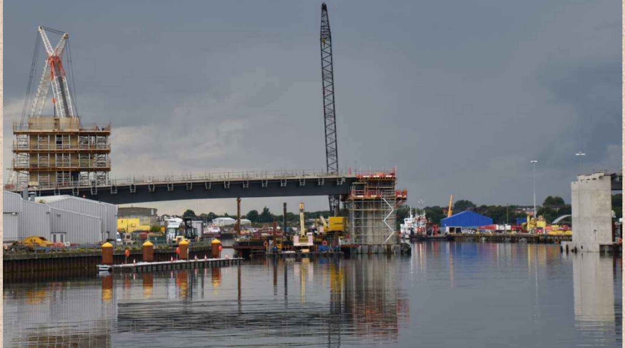
LW4 – Gull Wing Bridge South
